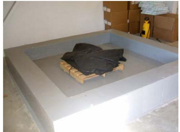
**This secondary containment area was designed and built for Ring Container in Sydney, Ohio. An additional containment area is in the works, which will be used in the quality control process and will require very strict and precise design requirements on the part of Scioto associates.**
